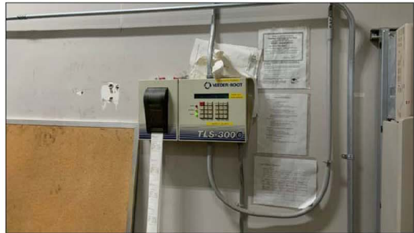
REMOVE VEEDER ROOT MONITOR AND LEAVE WITH COLLEGE. CAP ELECTRICAL CONDUIT.
