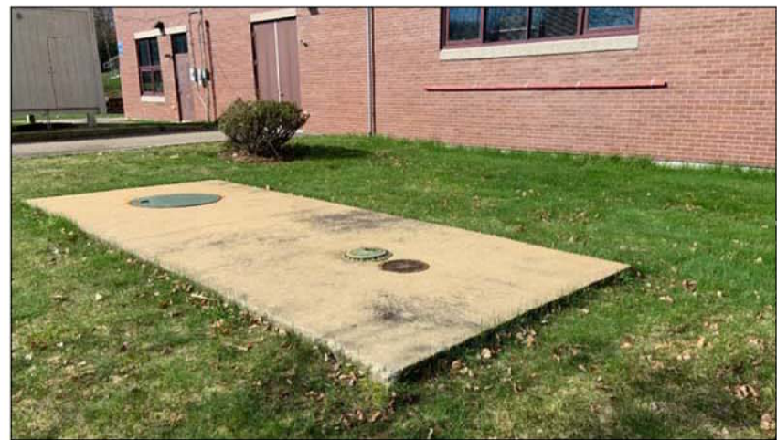
REMOVE AND DISPOSE OF 10,000 GALLON TANK AND CONCRETE PAD, PATCH THE DISTURBED GRASS AREA PER DETAIL. REMOVE AND DISPOSE OF VENT ON BUILDING EXTERIOR.
