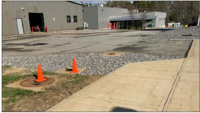
REMOVE AND DISPOSE OF 15,000 GALLON TANK PATCH ANY DISTURBED CONCRETE WALKWAY AND ADD NEW ADDITIONAL WALKWAY PER DETAIL, APPROX. 200 SF. REMOVE AND DISPOSE OF VENT ON BUILDING EXTERIOR.
