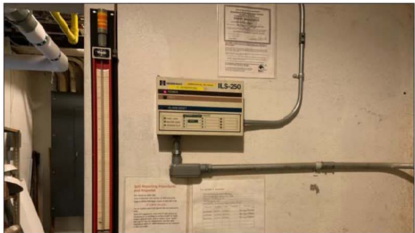
REMOVE VEEDER ROOT MONITOR AND LEAVE WITH COLLEGE. CAP ELECTRICAL CONDUIT.
