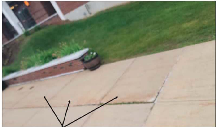
REMOVE AND REPLACE CONCRETE SQUARES. DOWEL INTO THE EXISTING TO STOP THE LIFTING. WIRE MESH TO BE ADDED.
