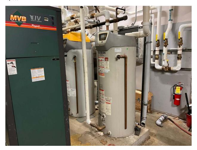
The Hot Water Tanks are currently fueled by natural gas. The photo below shows the piping and valve.
