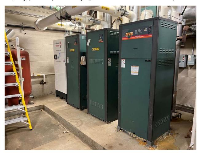
The boilers are currently fueled by natural gas. The photo below shows the piping and valve.
