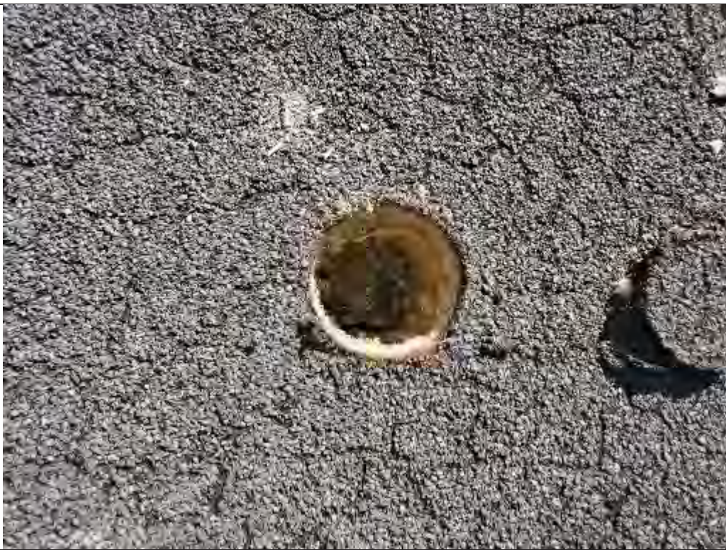
Typical core sample location showing roll asphalt roof on insulation on roof deck.
