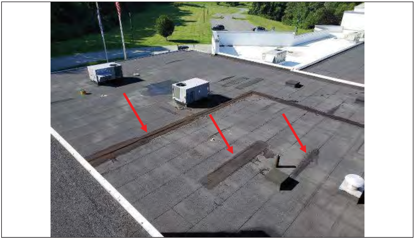
Variety of black roof patch materials throughout the roof. Homogeneous group determined to be ACM.
