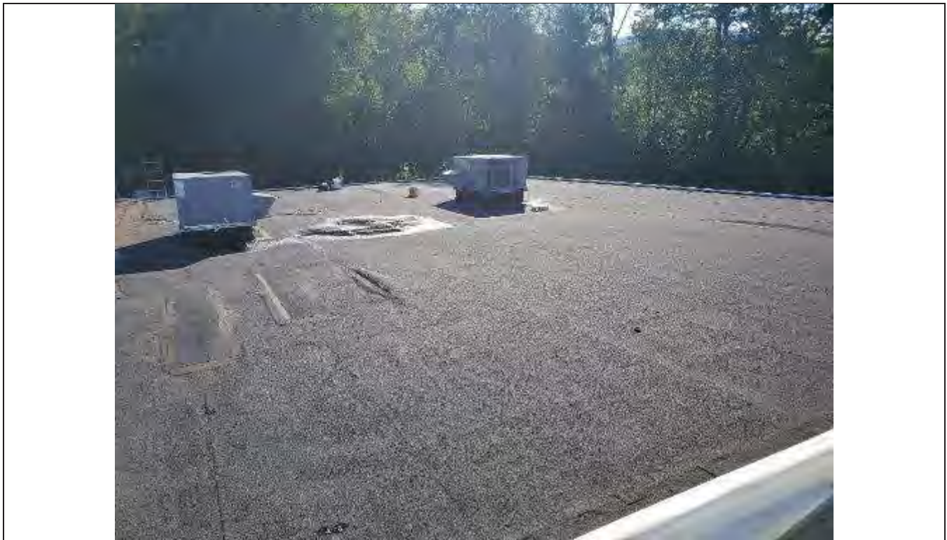
Rollled asphalt roofing present throughout roof. No asbestos detected directly associated with the roof itself.
